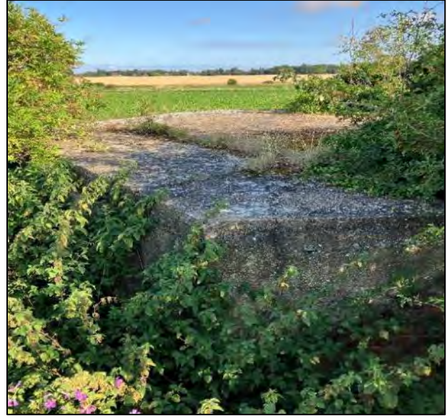
Figure 18: Roof of Defence
