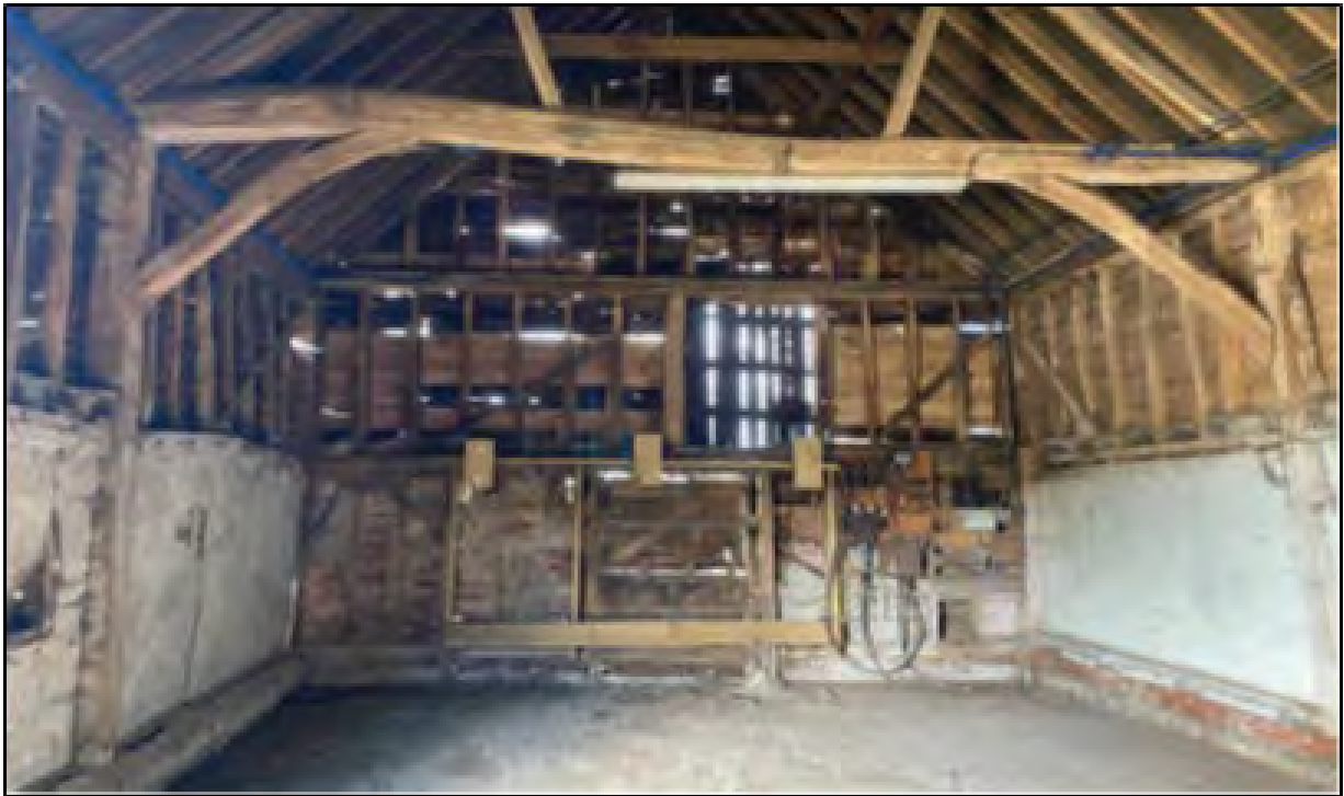
Figure 8: Alternative wall finishes in Barn attached to south of Big Black Barn
