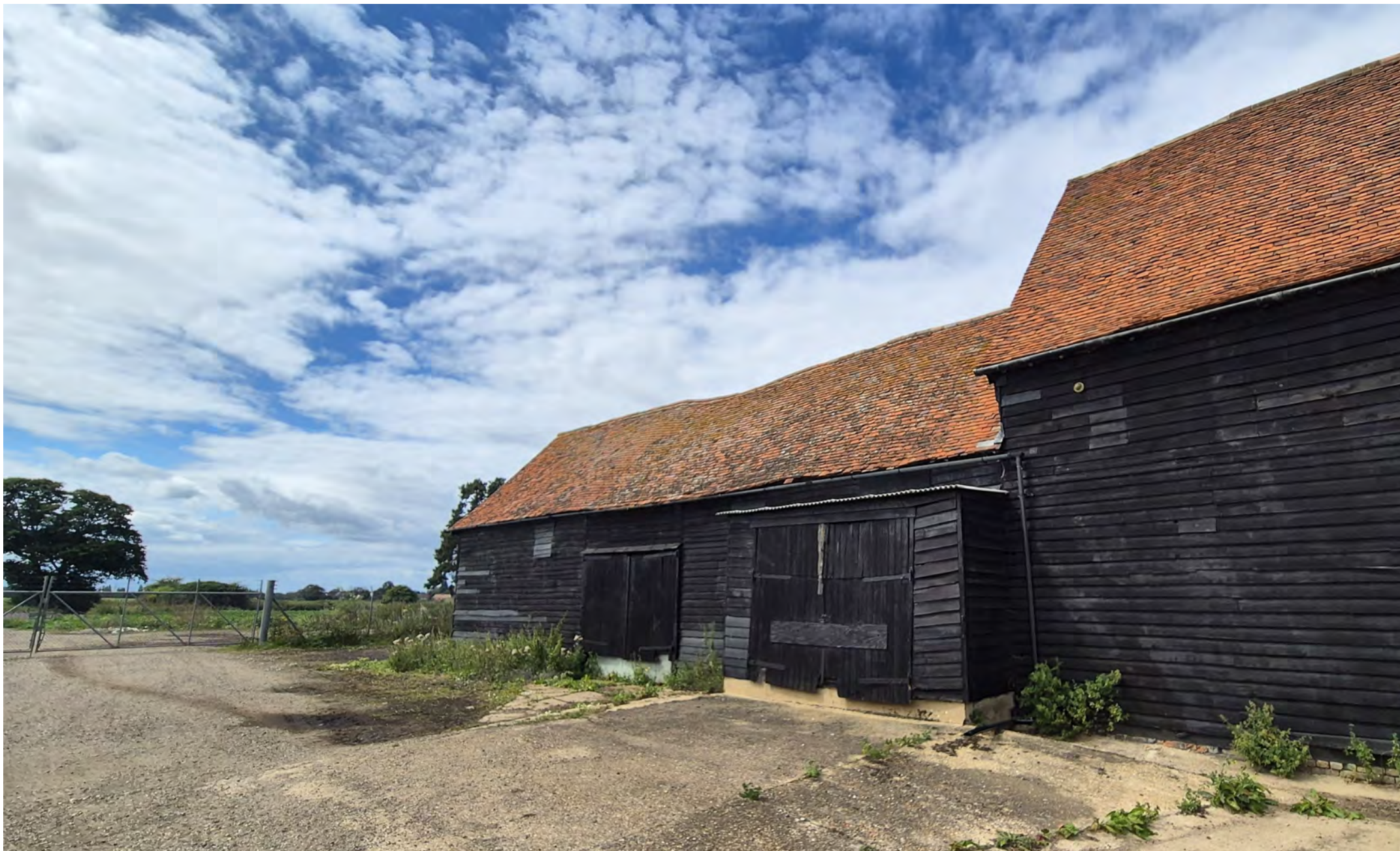
Eastern elevation of Big Black Barn
