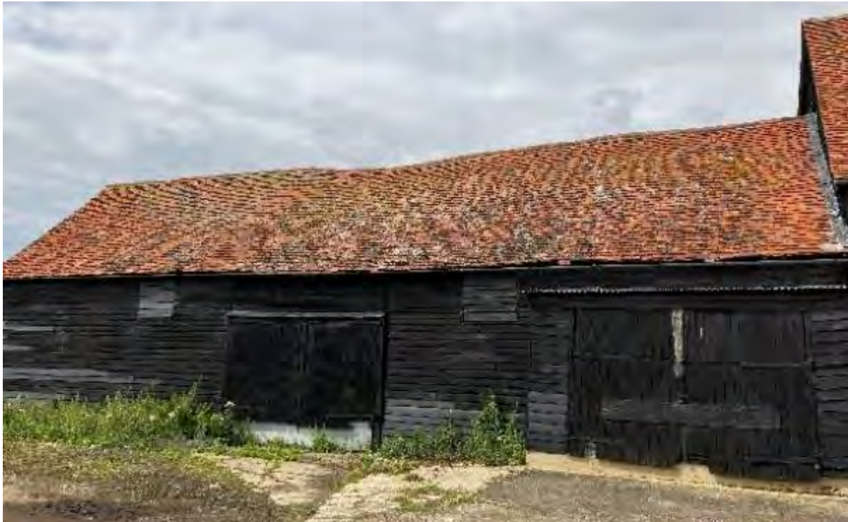
Figure 7: Exterior of Barn attached to south of Big Black Barn
