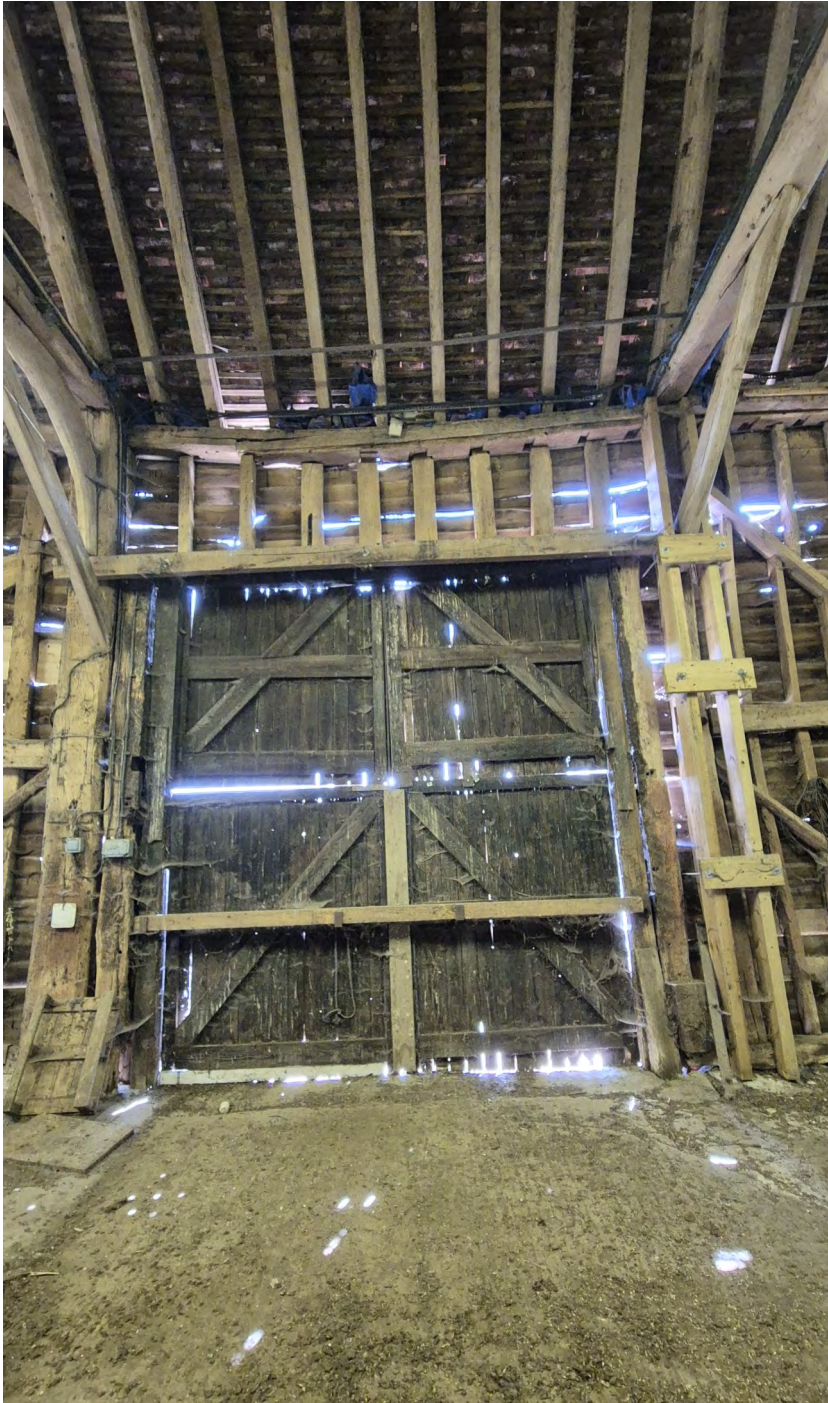
Big Black Barn - Bay 4 and 5 (Left: Eastern elevation / Right: Western elevation)
