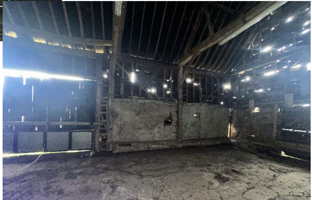
Below: Eastern Elevation internally (southern portion)
