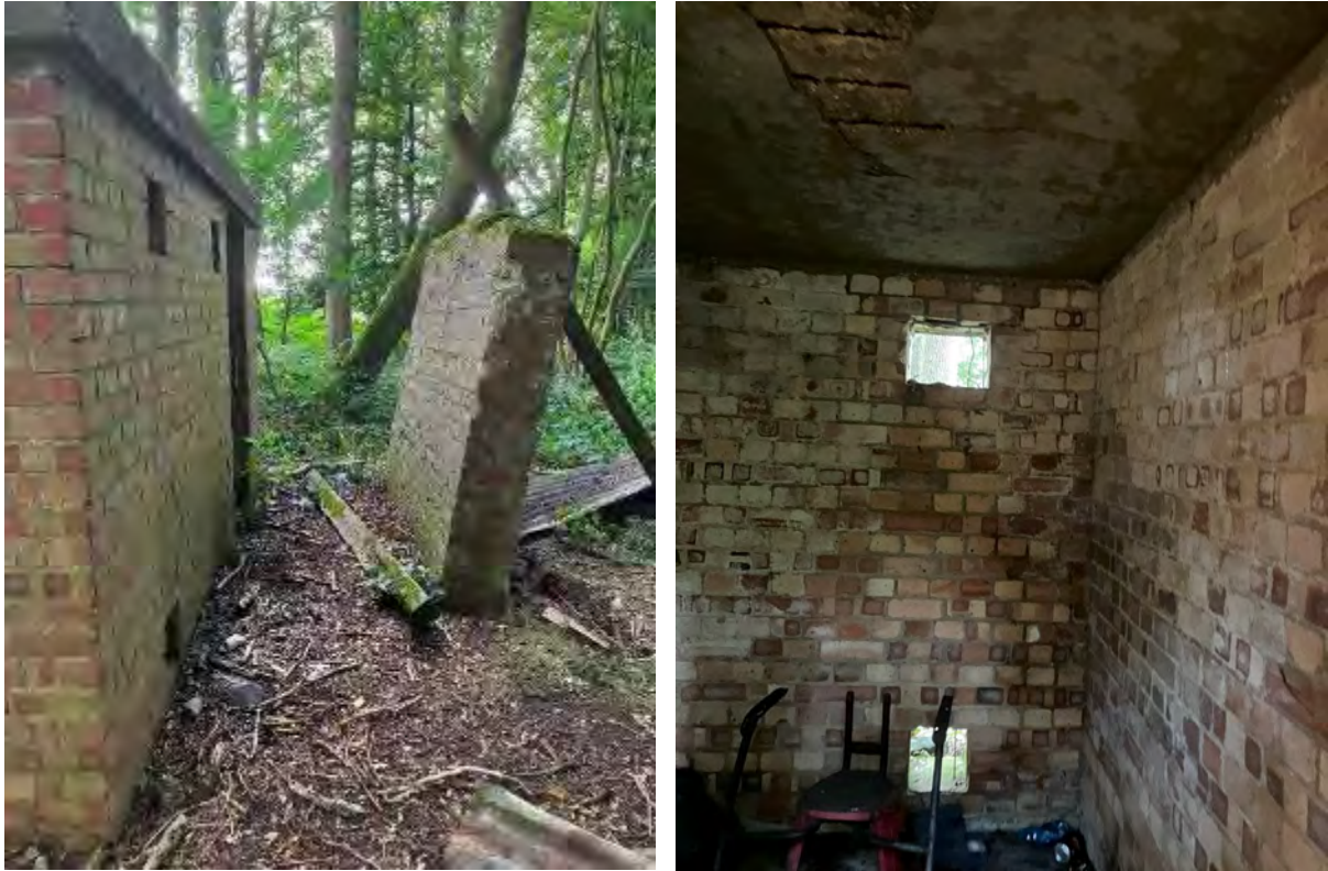
Figure 23: Ammunition store to pillbox 7 (Monument ID 13)
