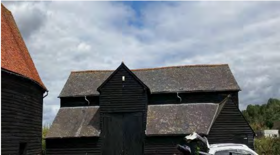
Figure 10 South elevation of Essex Barn:
