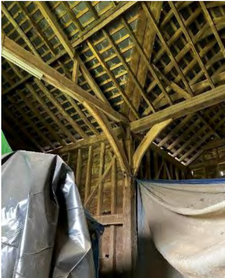
Figure 11: Internal roof detail - Essex Barn
