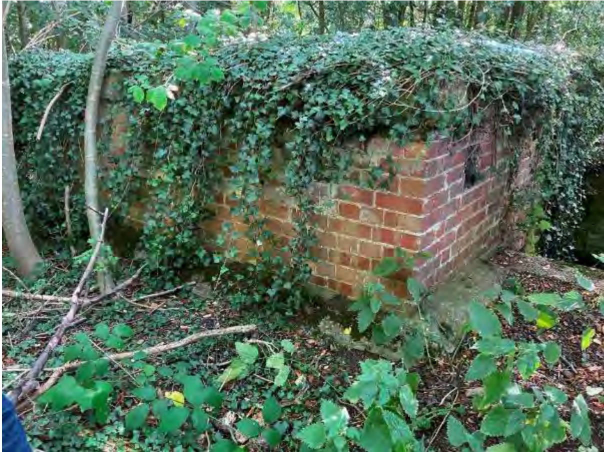
Figure 22: Ammunition store to pillbox 6 (Monument ID 11)
