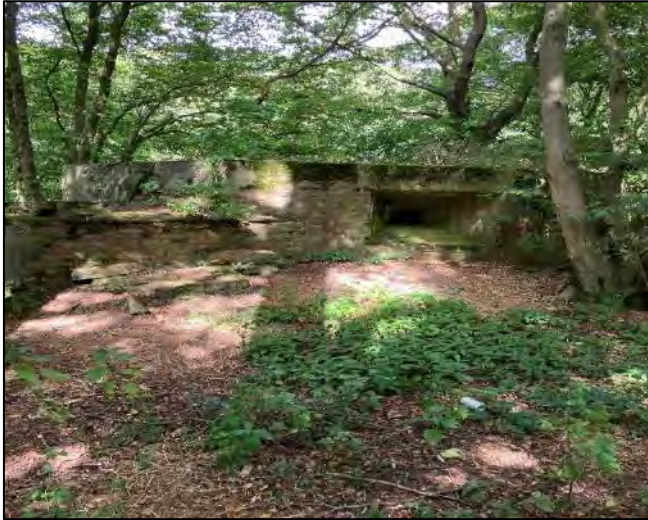
Figure 29: Roof of Defence
