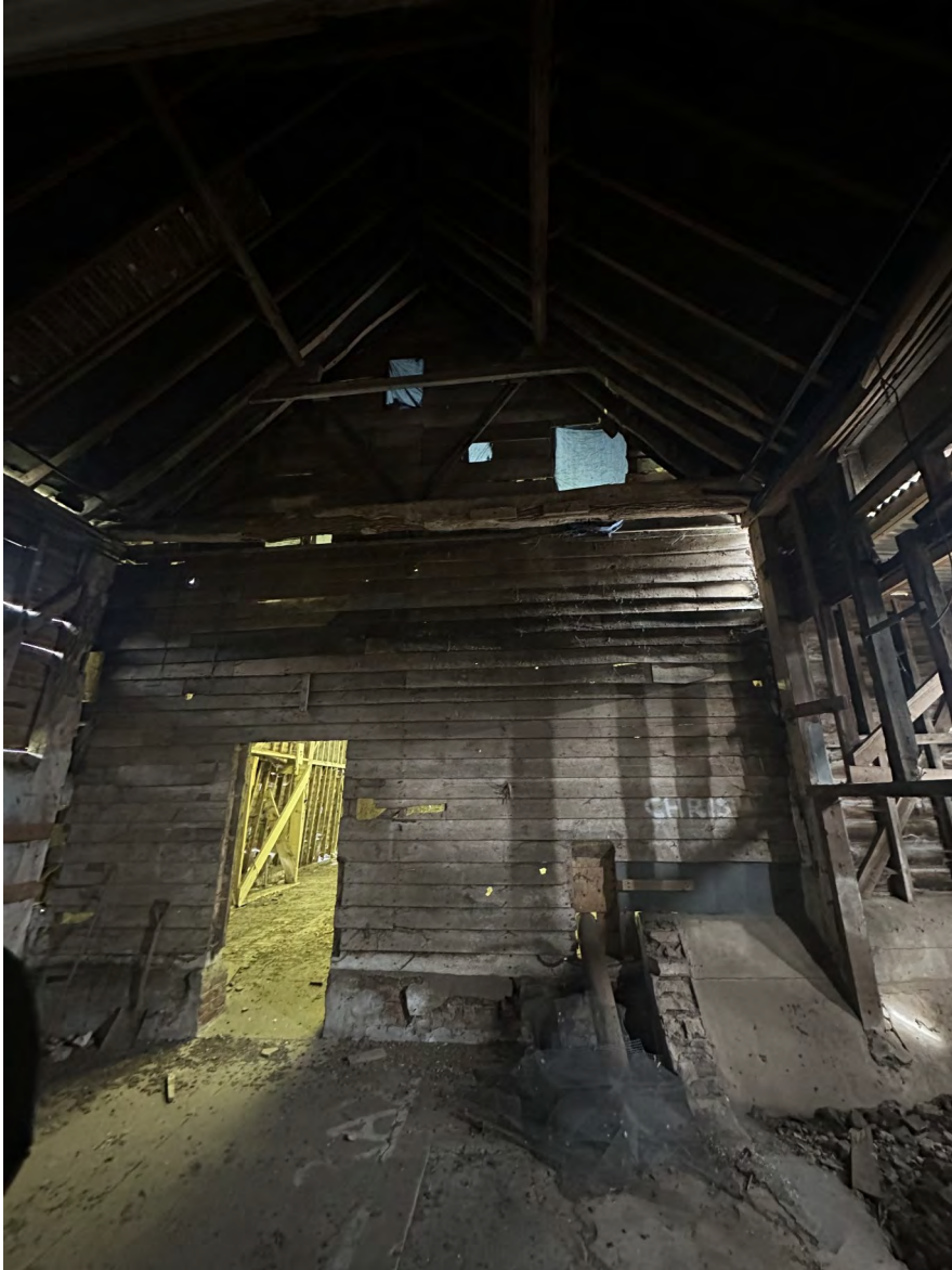
Northern gable (internal)
