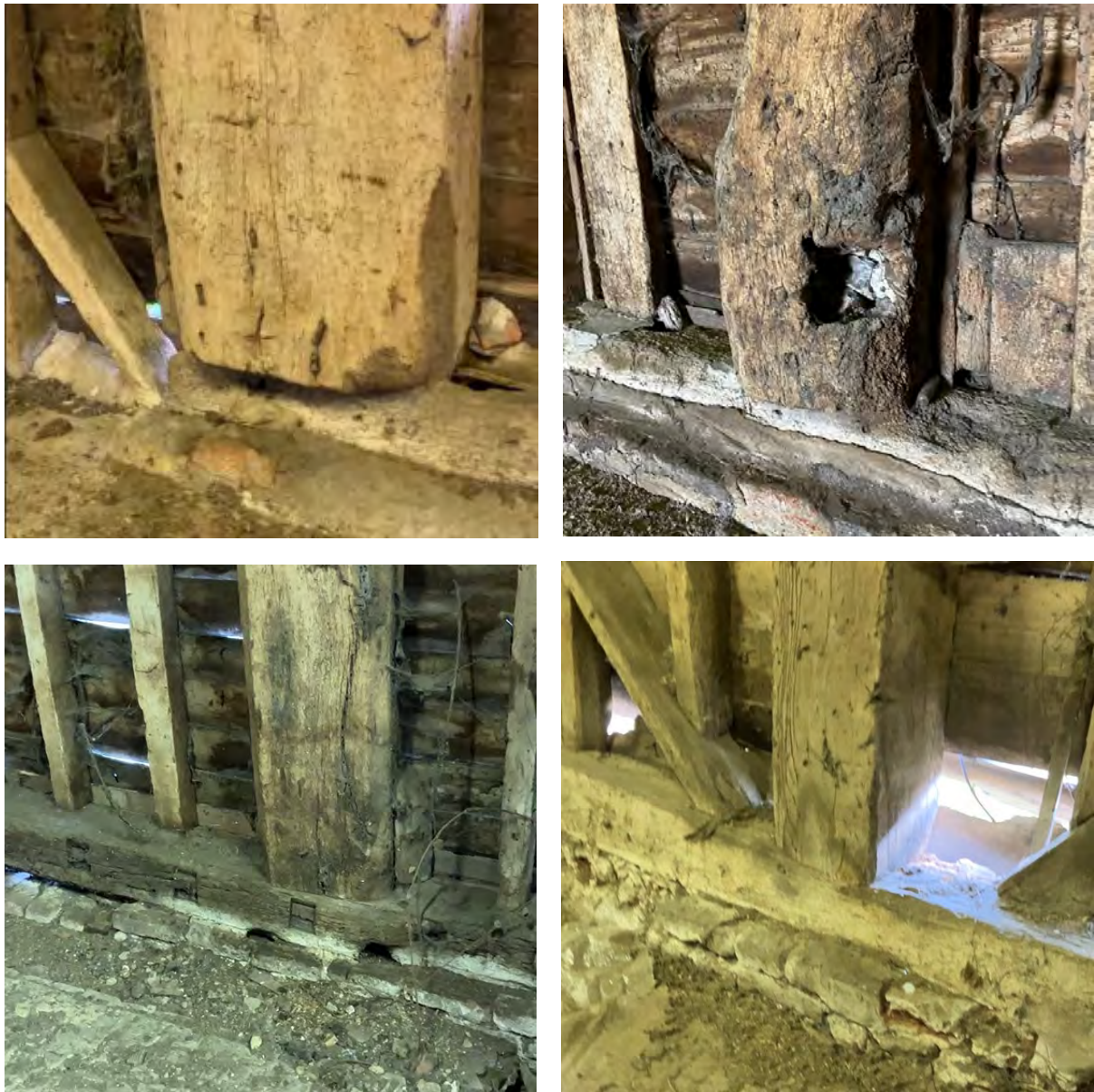
Figure 6: Black barn main post bases and sills
