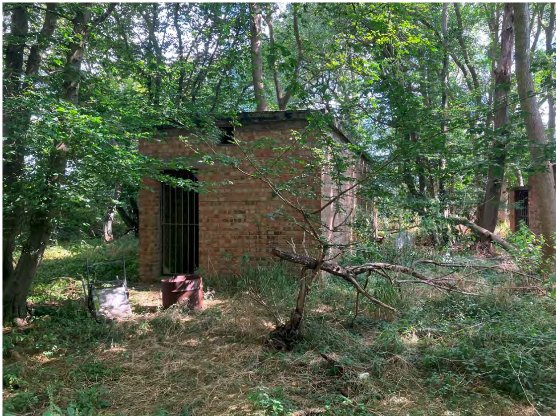
Monument 1: No.2 Sleeping Quarters building (Designation area 11) - External
