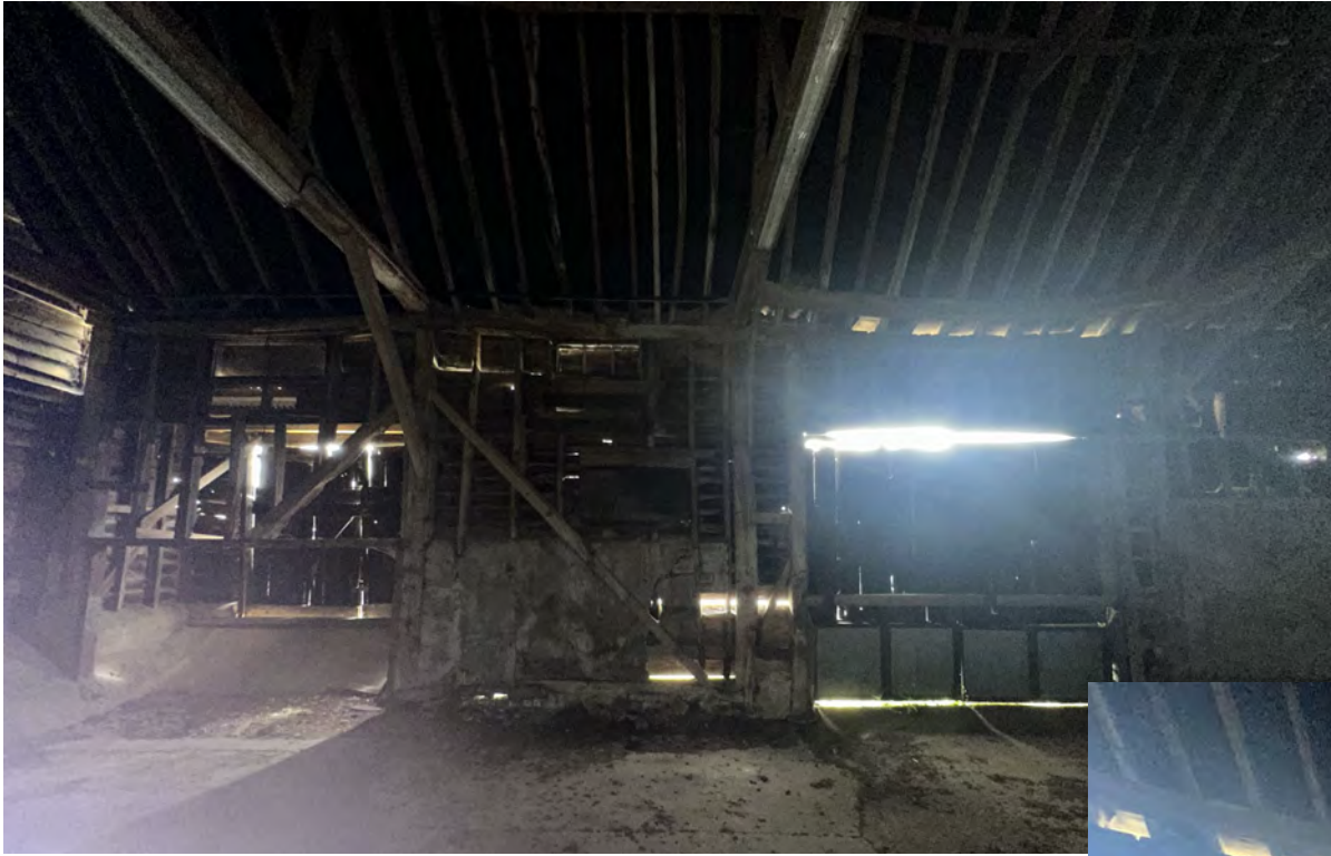
Above: Eastern Elevation internally (northern portion)
