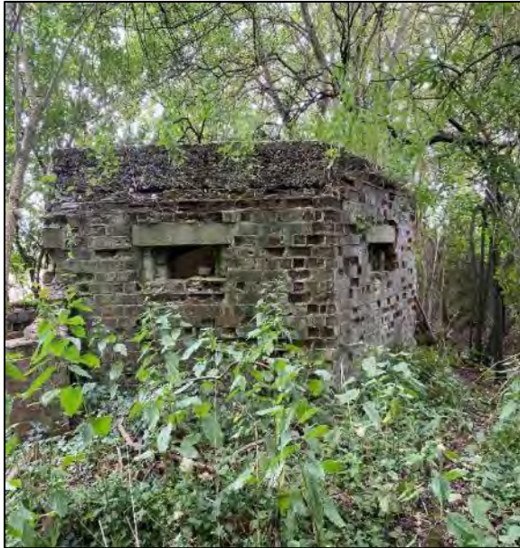
Figure 6: Brick Defence post
