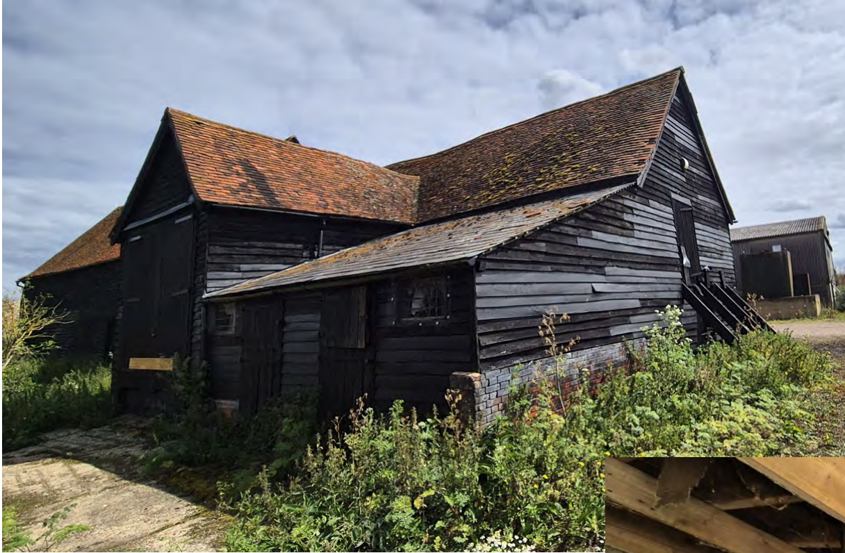
Exterior - lean-to stables to SW elevation
