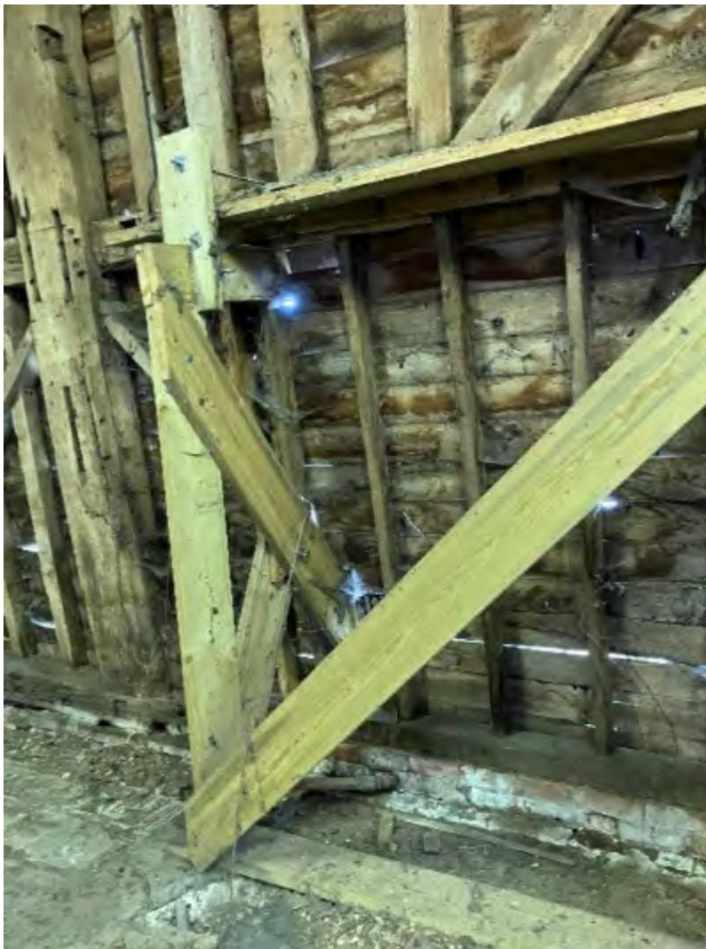
Figure 6: Internal Shoring
