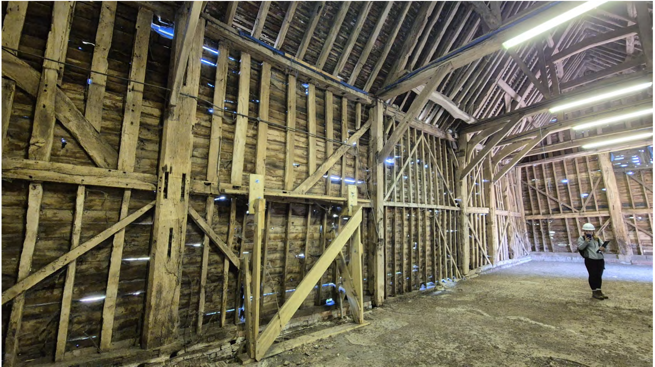
Western Elevation - Internal - Big Black Barn
