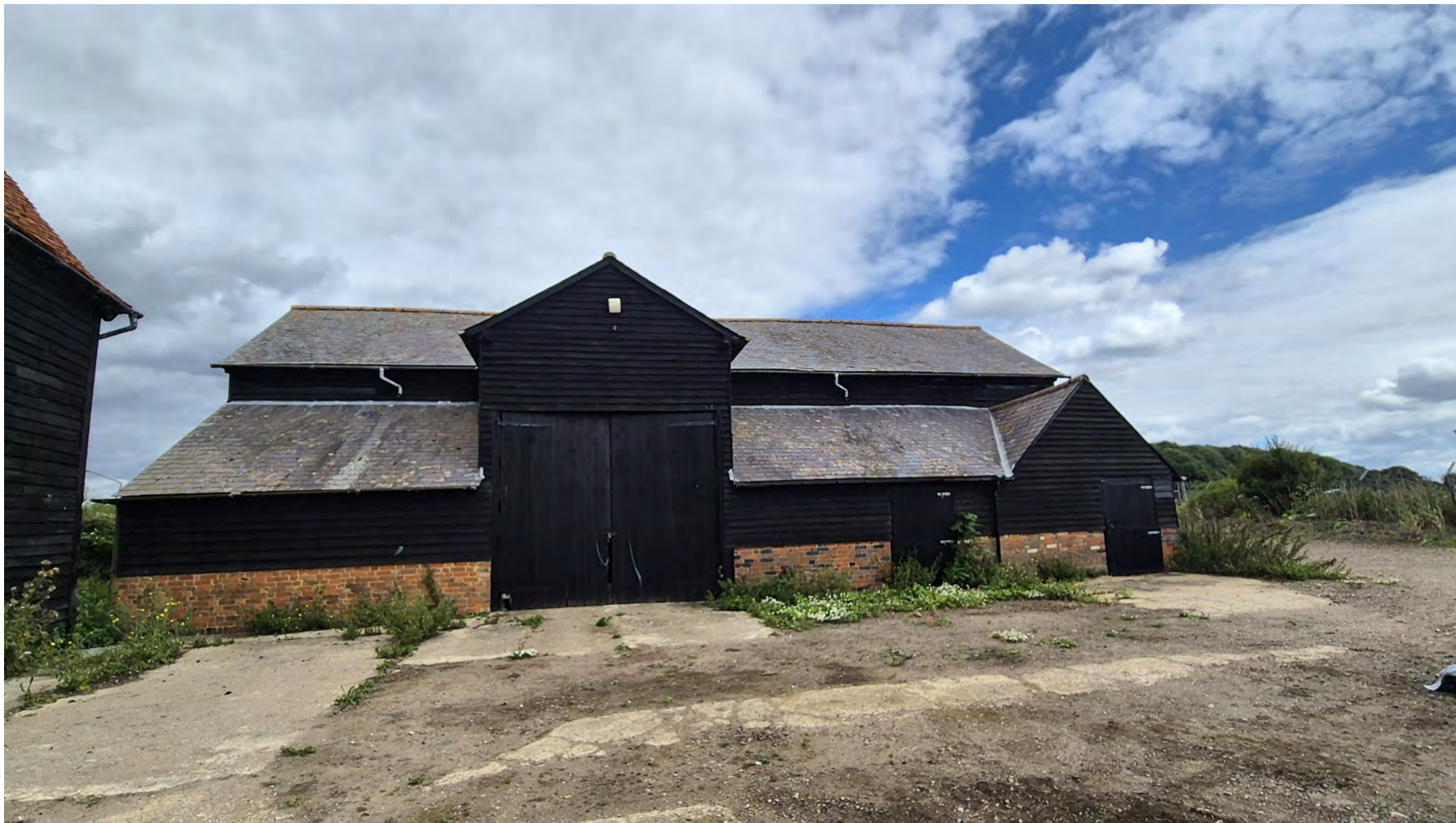
Southern elevation of Essex Barn
