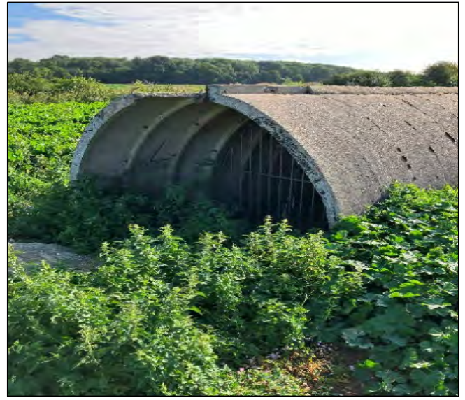
Figure 21: Escape Hatch on roof
