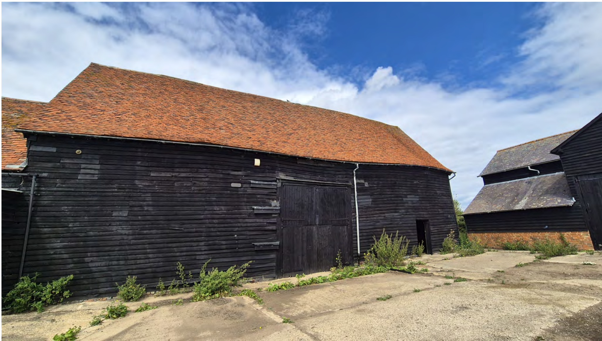
Eastern elevation of Big Black Barn
