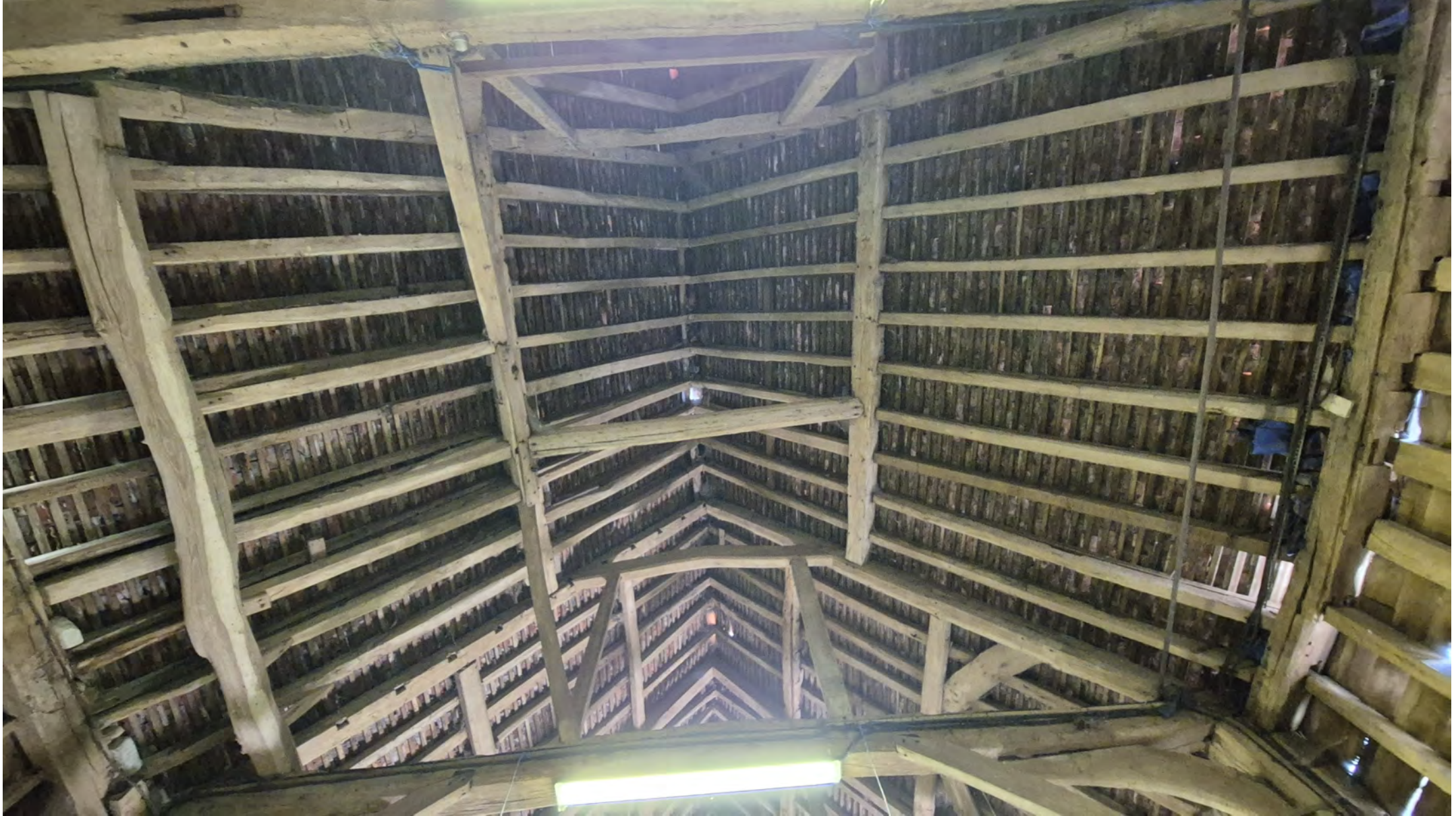
Big Black Barn - Bay 4 and 5 Roof Structure
