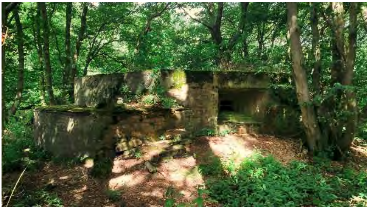
Figure 14: Typical hexagonal pillbox (No.7 – Monument ID 12)
