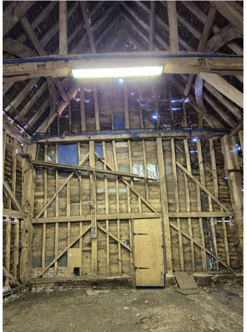
Southern elevation - Internal - Big Black Barn
