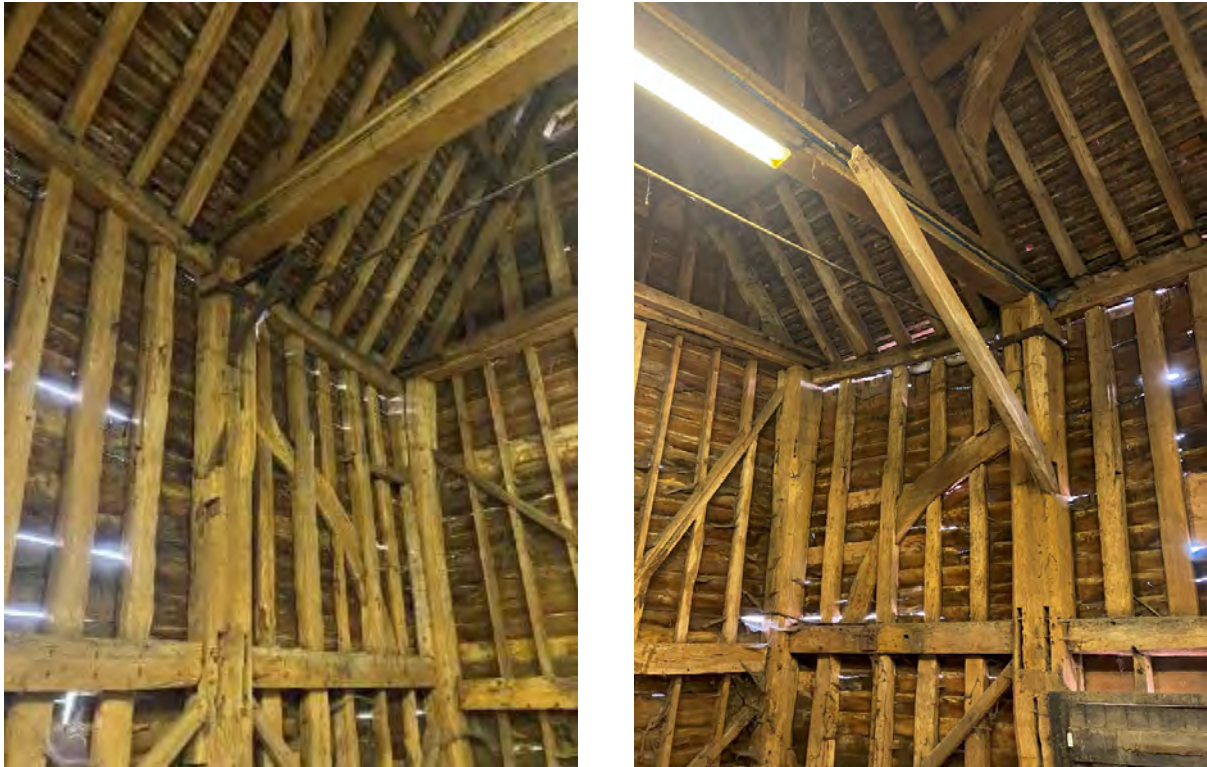
Figure 5: Black Barn eastern frame issues
