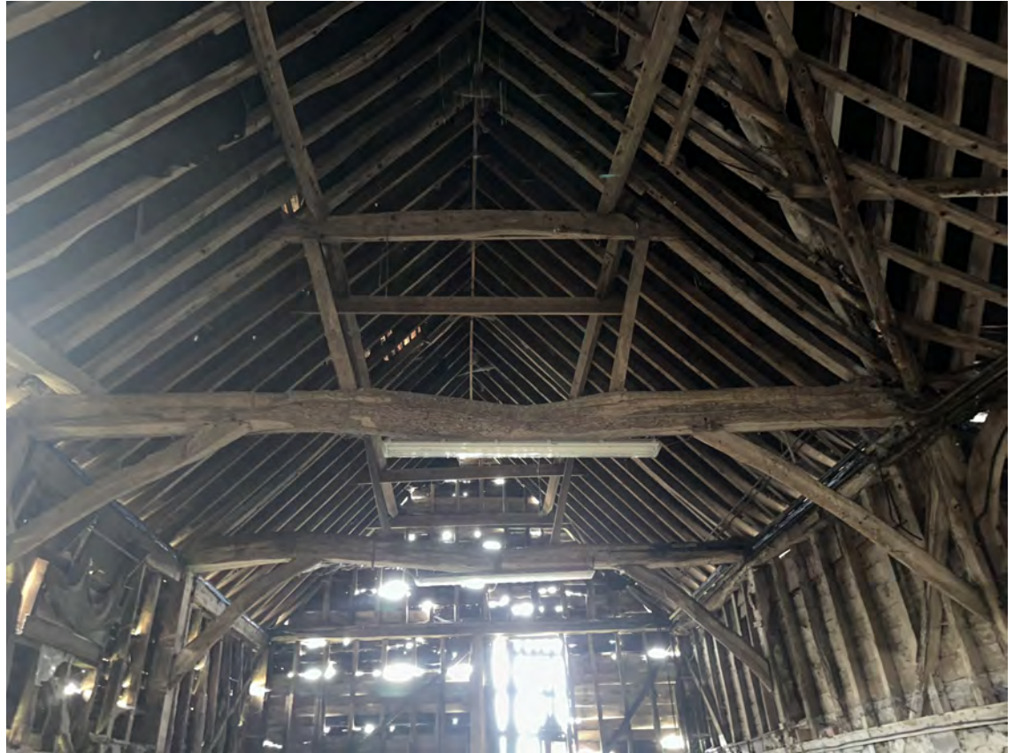
Roof structure (main barn)
