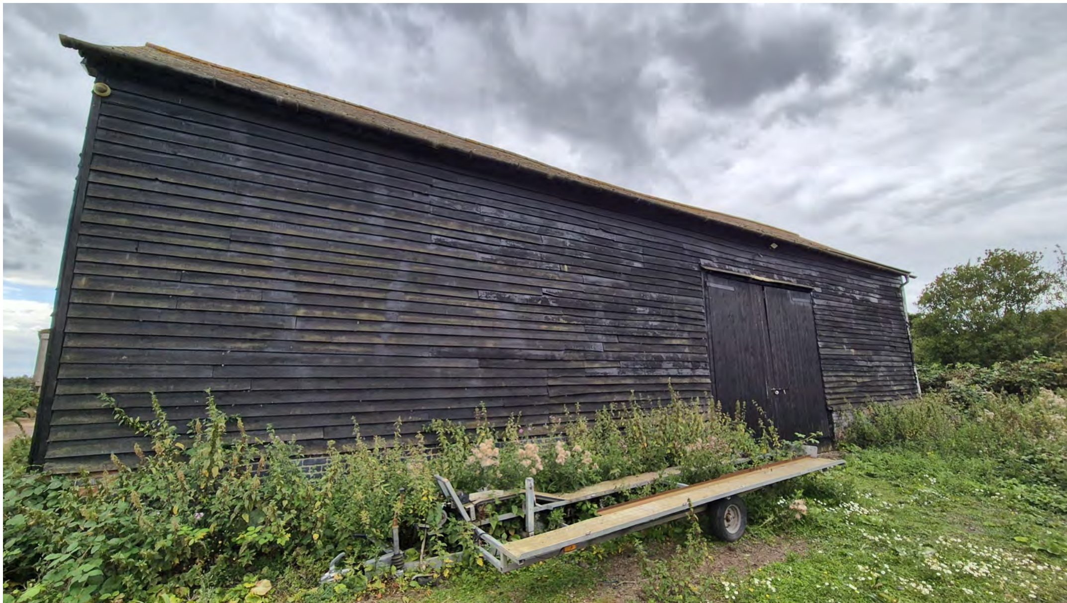
Northern elevation of Essex Barn
