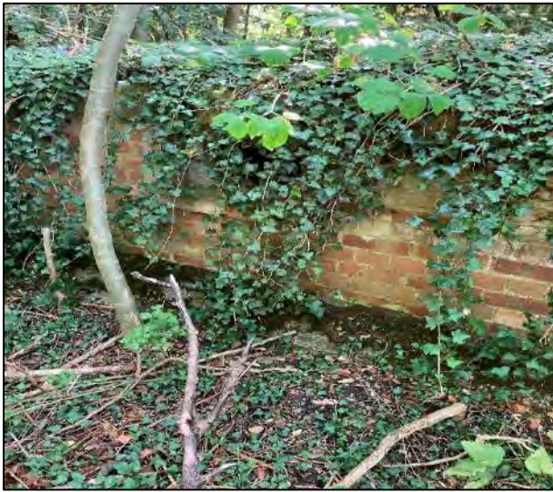
Figure 25: Brick Defence Post
